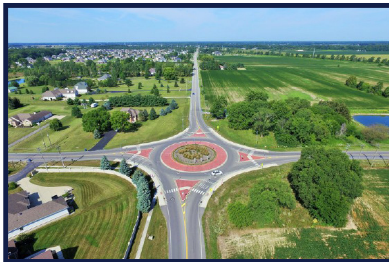
The Stitt Road and Waterville-Monclova Road intersection is a single-lane, all-way yield roundabout.
